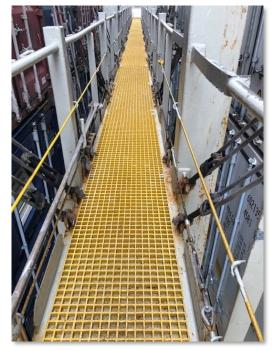
After trying several paint formulations, alternative protective solutions were installed such as fiberglass grating.
